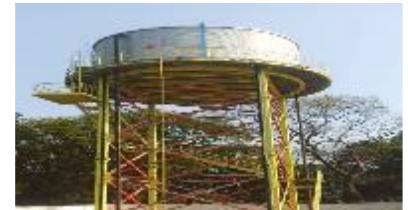
Water Tank, Uttar Pradesh
